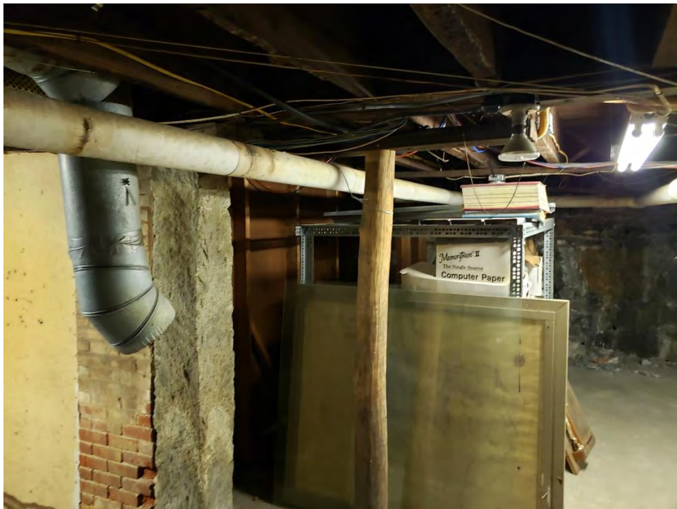
Photo 10: Basement Granite Columns and Timber Pole Reinforcing Supporting First Floor Framing
