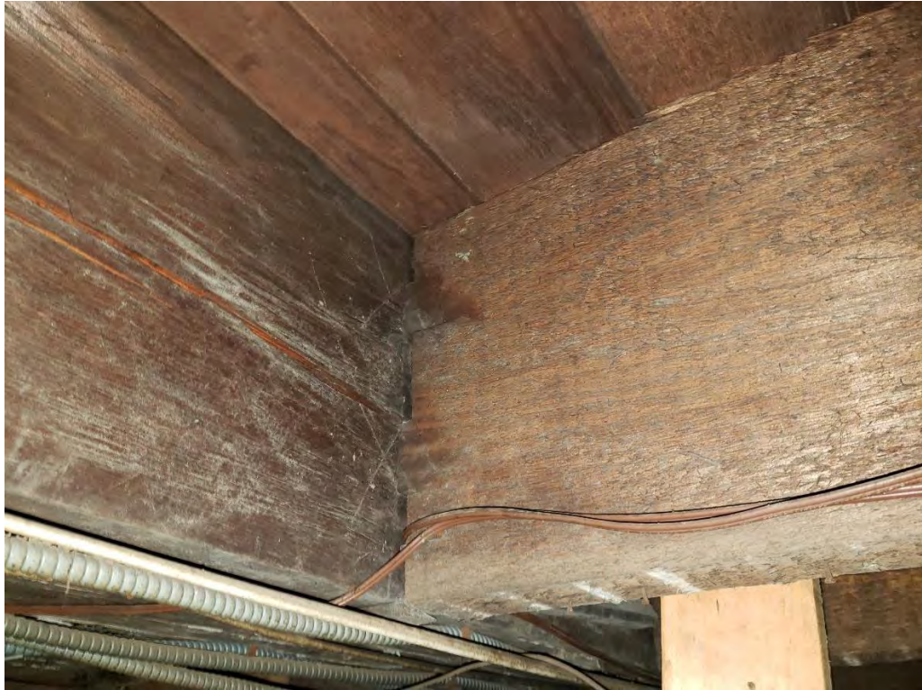
Photo 11: Typical Double Mortise Connection of First Floor Joists to Timber Girders
