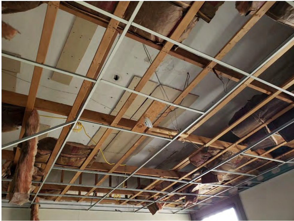
Photo 9: Second Level Ceiling Attached to Attic Framing
