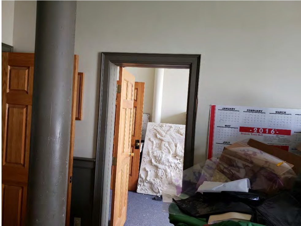
Photo 3: Round Wood Pole Columns Supporting Second Floor Framing
