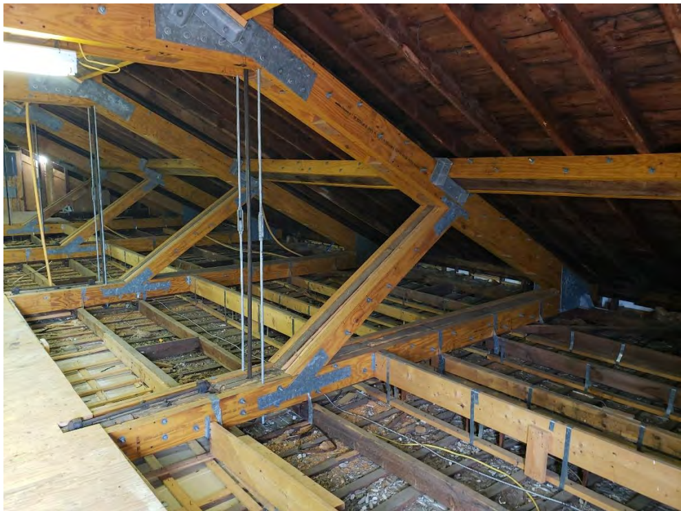
Photo 4: Reinforced Roof Trusses and Roof Framing in Attic
